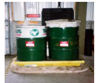
Mercury waste storage containers with spill containment trays placed below (UNDP-GEF)
